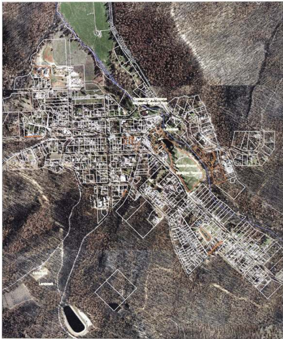
Marysville - Post Fire Aerial Photography
